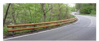
Shinshu-type wooden guardrails were developed jointly by local contractors, logging companies and the civil engineering department of the prefectural government. The guardrails are as durable as those made of steel, and created 5 times the number of local jobs with the same budget.
